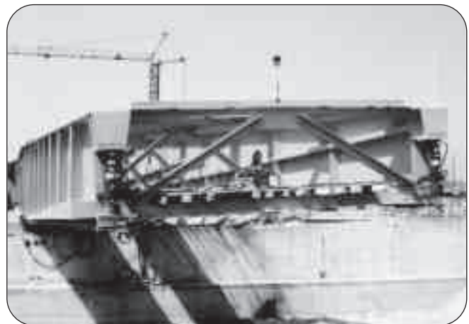
Launching-nose lifting unit hydraulic lifting unit bolted to nose.
