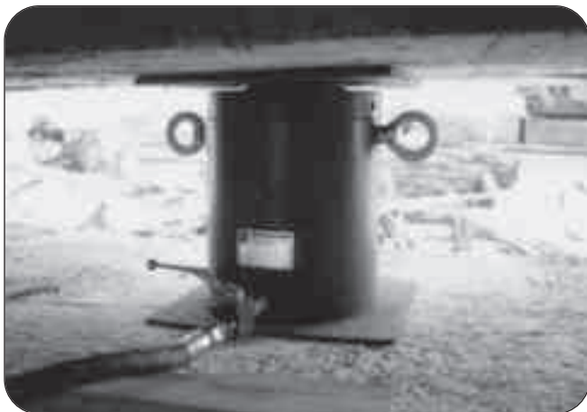
Hydraulic jack with adjustable locking ring.
